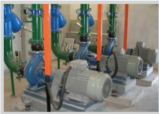
EUROFLO End Suction Pumpset used in HVAC and cooling tower system for commercial building.
